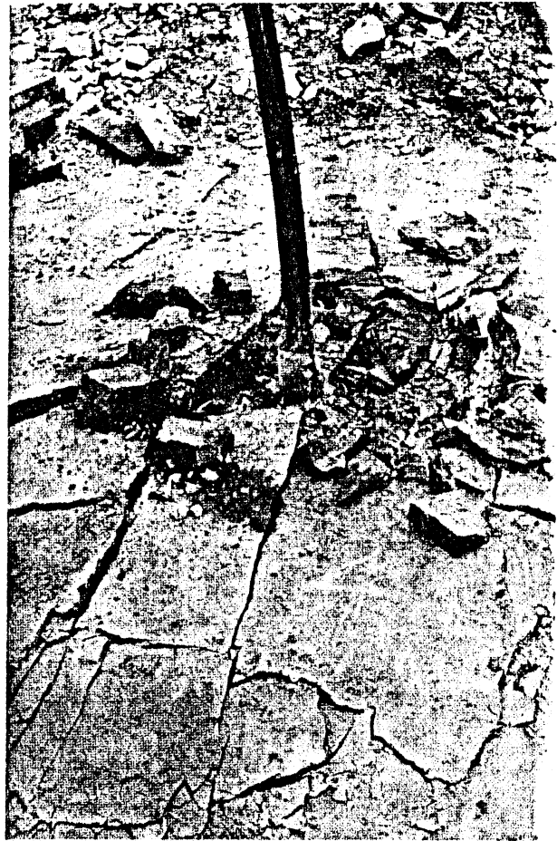
Fig. 2. — Failure volume induced at anchor 4, showing the control of the dominant NW-SE joints.
