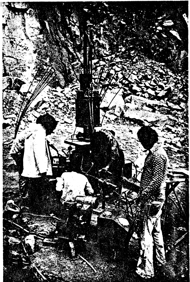
Testing of ground anchors in Britain
