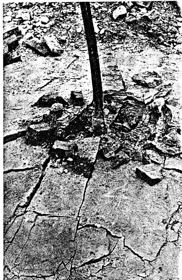
Fig. 2. — Failure volume induced at anchor 4, showing the control of the dominant NW-SE joints.
