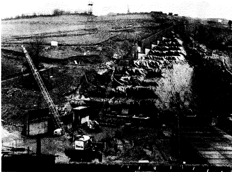
Fig 5. Rock exposed on south side, under buttresses 14-16.
