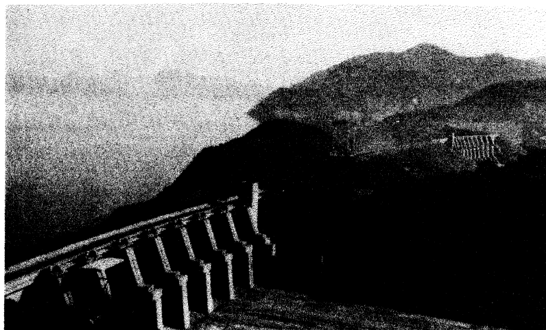
Fig. 2. General view of service spillway gates (foreground), Auxiliary Dam 2, auxiliary spillway gates, and the curved Auxiliary Dam 1, right
