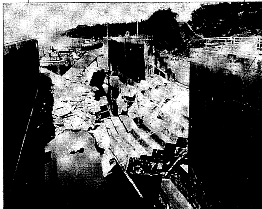
IN 1961, WORKERS TRIED TO INCORPORATE AN EXISTING LOCK WALL INTO A NEW COFFERDAM. A MAJOR PORTION OF THE LAND WALL SLID INTO DEWATERED EXCAVATION KILLING SEVERAL PEOPLE.
