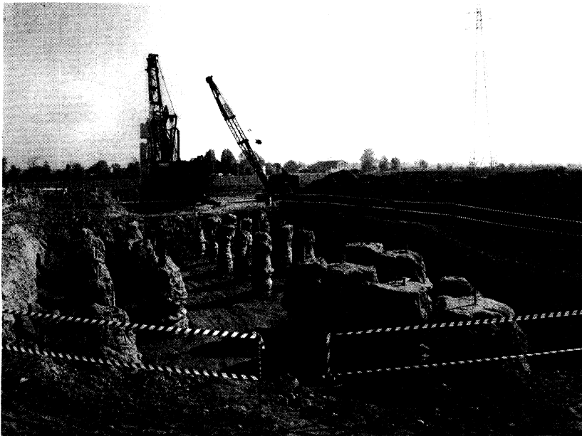
Photograph 1. Excavated test columns created by one fluid (back center), two fluid (left) and three fluid (right front) systems. Courtesy of Rodio, Milan.
