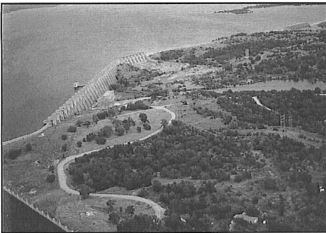
Figure 2 – Aerial view of Buchanan Dam
