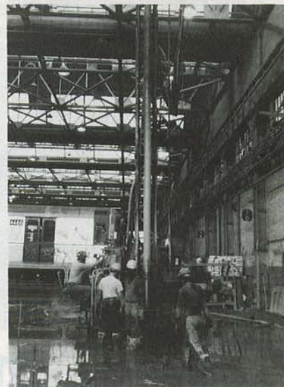
Fig. 4. Standard diesel hydraulic drill rig. Coney Island, NY.
