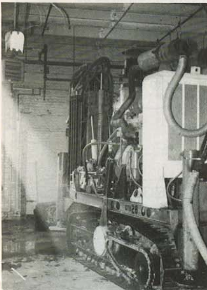
Fig. 3. Special low headroom drilling equipment (8' mast). Coney Island, NY.
