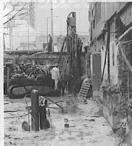
Fig. 1. Typical minipile installation conditions. Boylston St. Boston, MA.
