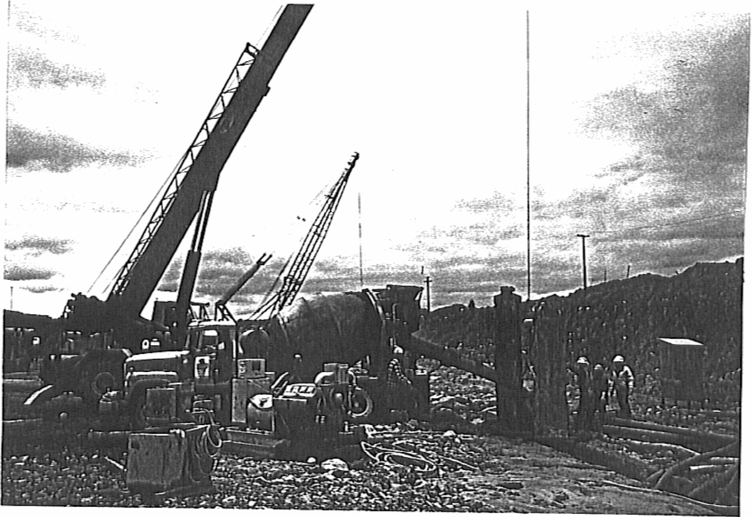
Photograph 5. Concreting of Primary panel with two end stops in place.
