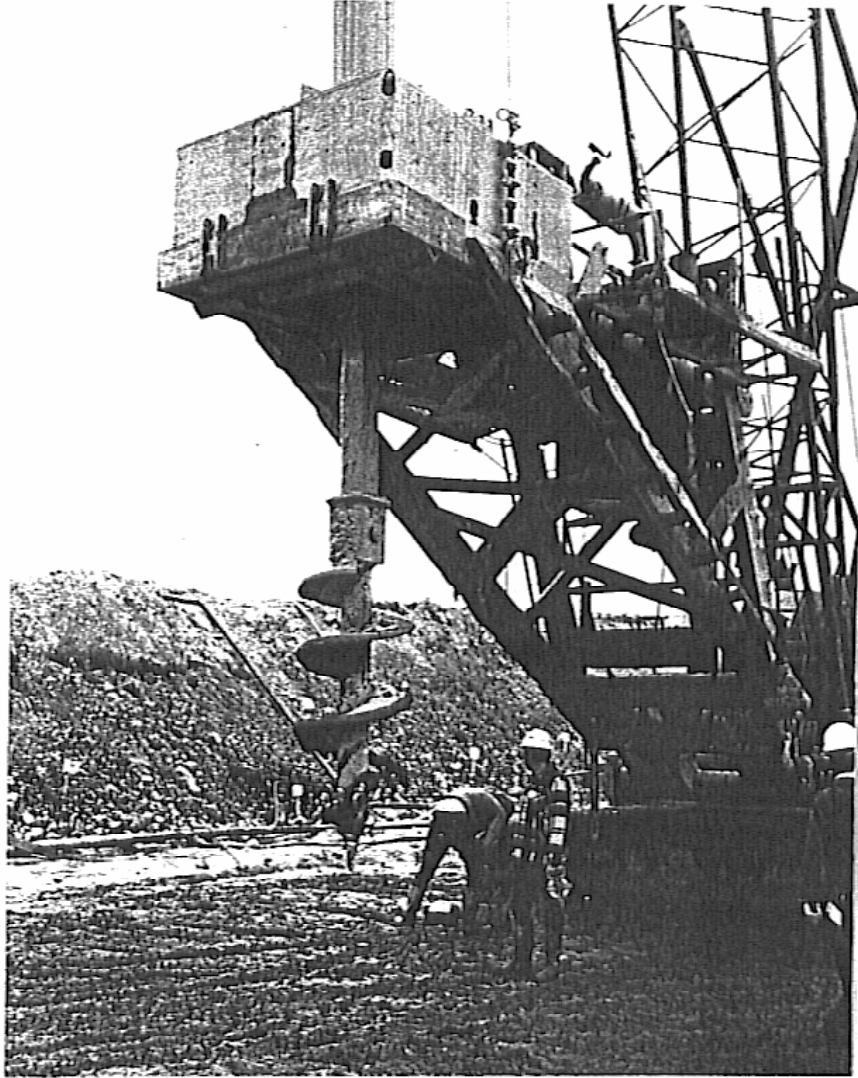
Photograph 3. Large diameter auger used to predrill through the till.
