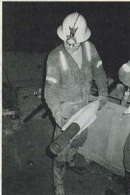
Photograph 1: Fitting fabric bag over plastic MPSP.
