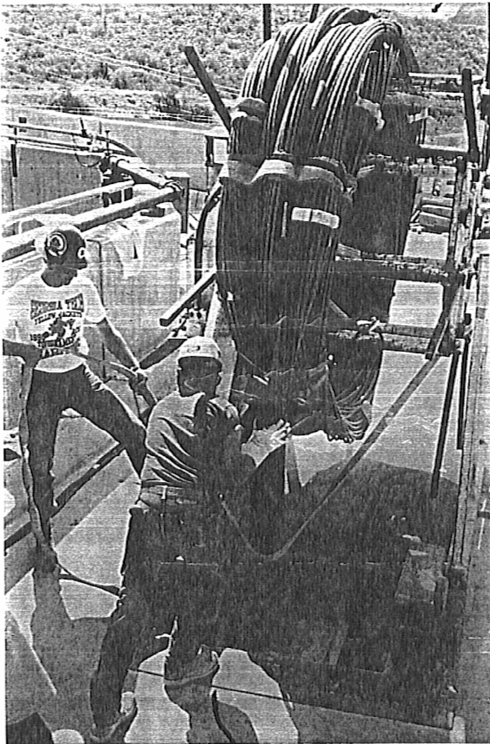
Figure 4. Photograph of tendon uncoiler
