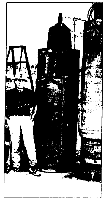
Drill piling tools.
